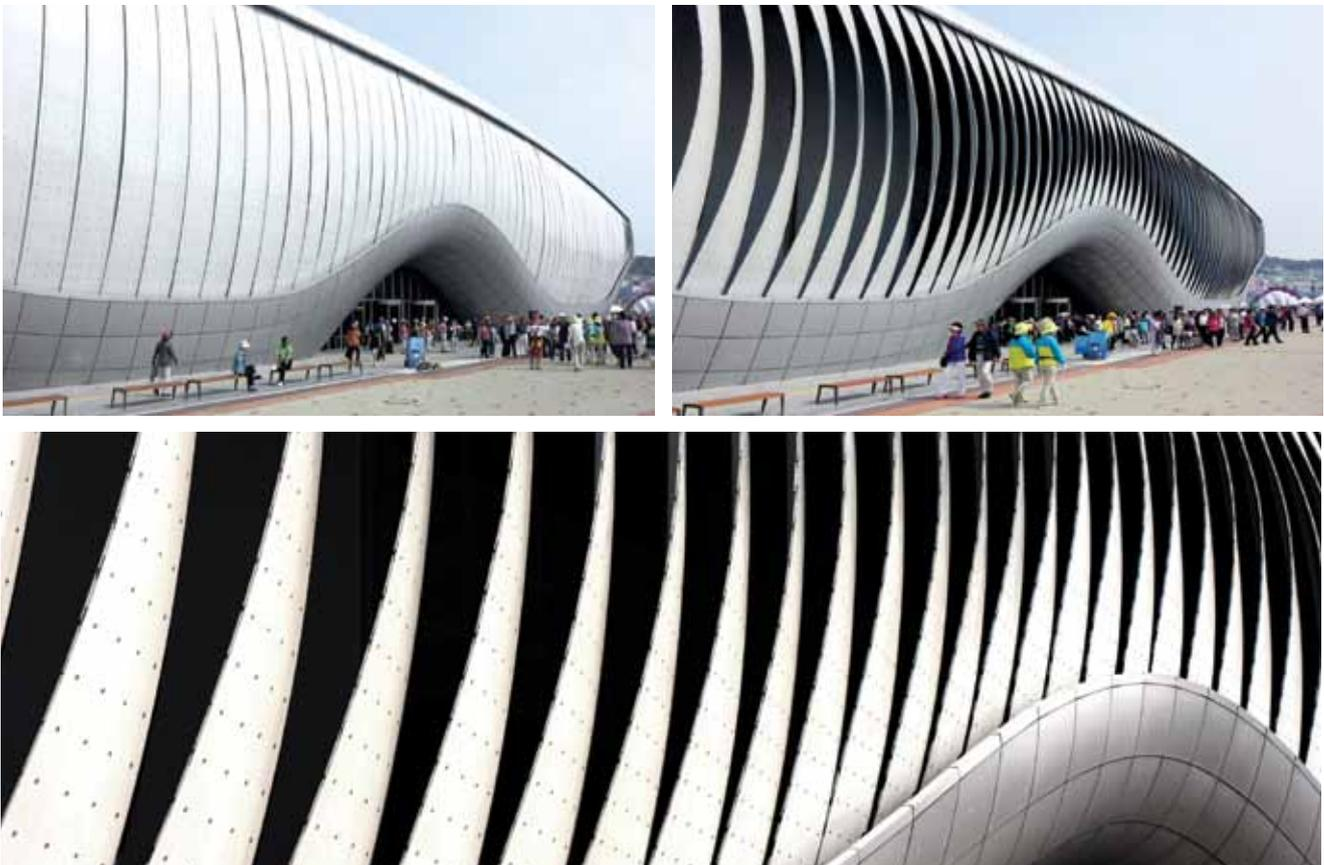
Fig.22-24: Kinematic facade of the Thematic Pavilion EXPO 2012 in Yeosu, South-Korea. Architects: soma-architecture, Vienna; Engineer for Kinetic Facade: Knippers Helbig, Stuttgart, New York.
